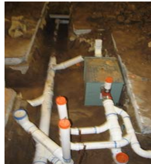
Plumbing/grease trap
